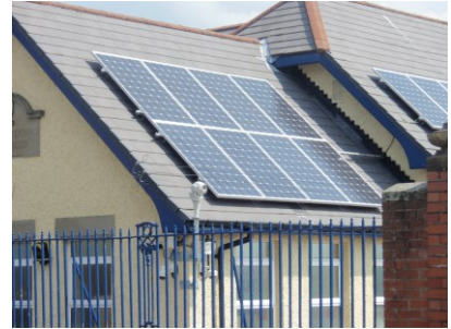
83 - Solar panels at Park Primary School
