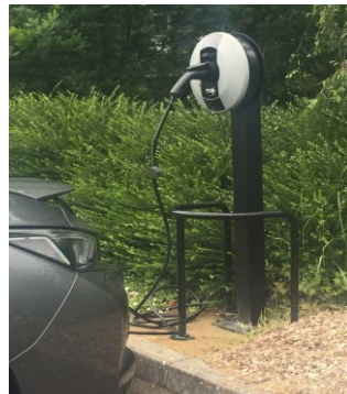
88 - Electric vehicle charge point at Penallta House
