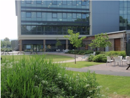
84 - Outside area at Penallta House
